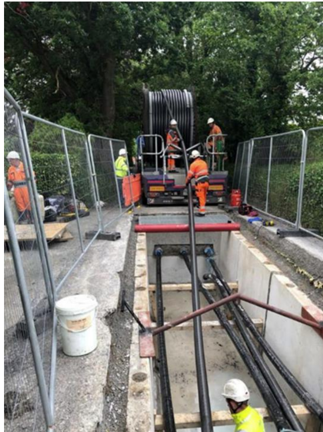
Figure 2.5: Typical Set-Up of HV Cable Pulling Procedure
